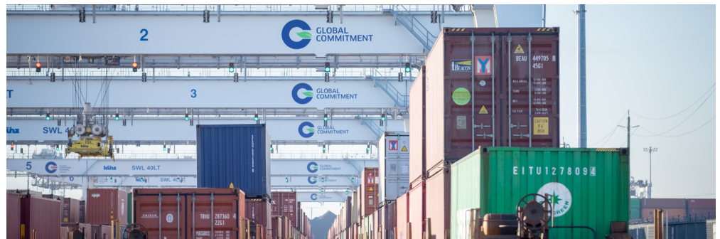
GCT Deltaport: Electric Cantilevered Rail Mounted Gantry cranes
